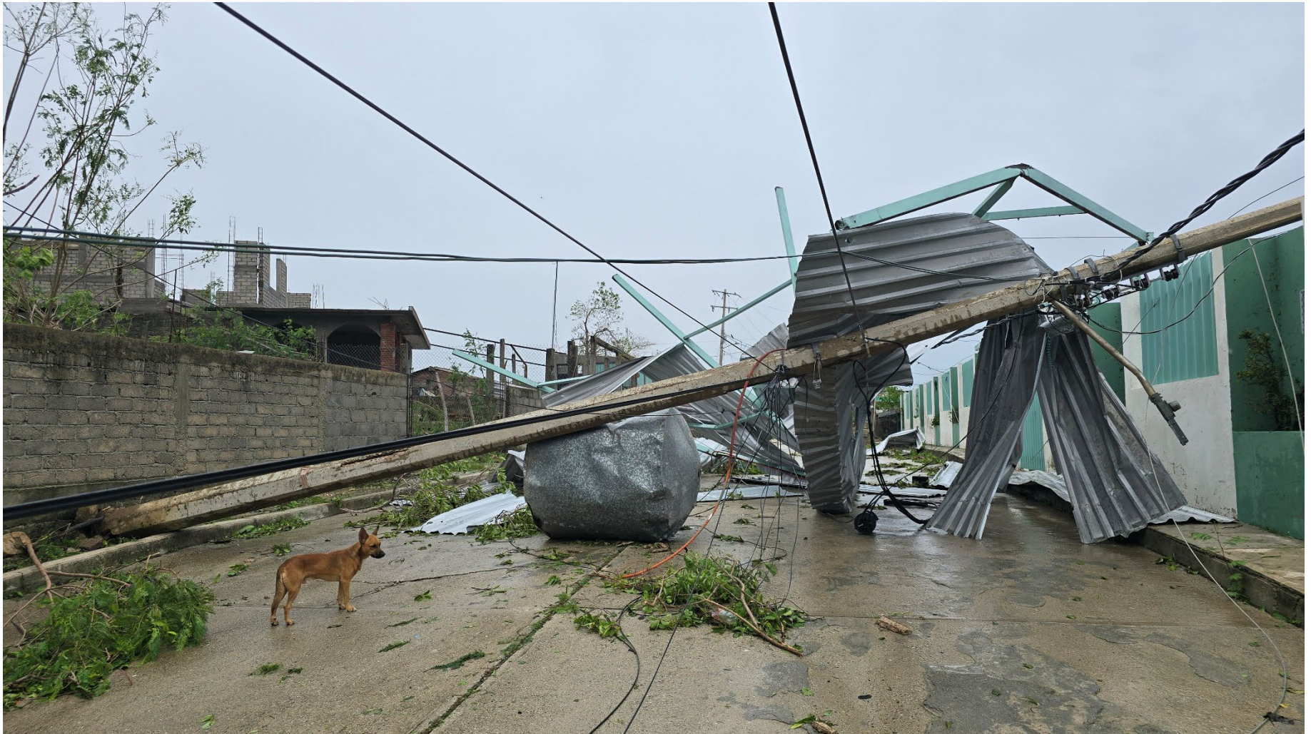
Figure 12. A utility poll knocked down along with other debris in San Jose Estancia Grande, Mexico following the landfall of Hurricane Erick. Image courtesy of Josh Morgerman, iCyclone.
