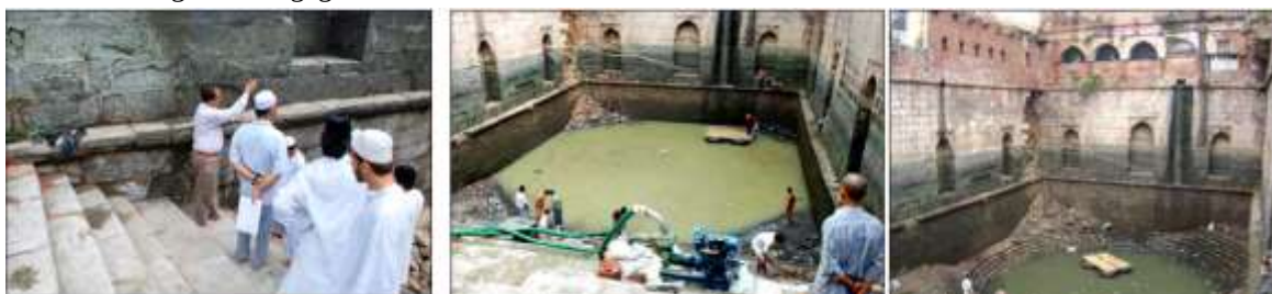
Fig no. 18, 19 &amp; 20 Ongoing projects of AConservation of stepwell of Hazrat Nizamuddin Baoli
