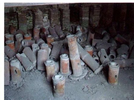
Fig. 20. Varna (Odessos): The Roman civic baths. Hypocaust, showing the use of vertical clay pipes used in two interlocking sections to support the suspended floor and convey heat. Late second century AD.
