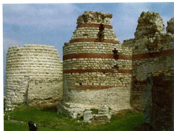
Fig. 15. Nessebar ( Mesembria Pontica ): Exterior view of the Early Byzantine fortifications just north of the west gate, looking north, showing two U-shaped towers using opus mixtum and ashlar construction techniques. Fifth to sixth centuries AD onwards. Photo: © Grahame Soffe.
