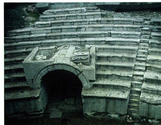
Fig. 2. Plovdiv (Philippopolis/Trimontium): Stadium or circus, north end of the arena, 70m wide, with marble seating showing sculptured 'legs' and a vaulted and arched main(?) entrance. Fragment of architrave with motifs of bucrania linked by garlands, interspersed with masks and rosettes. Photo: © Grahame Soffe.
