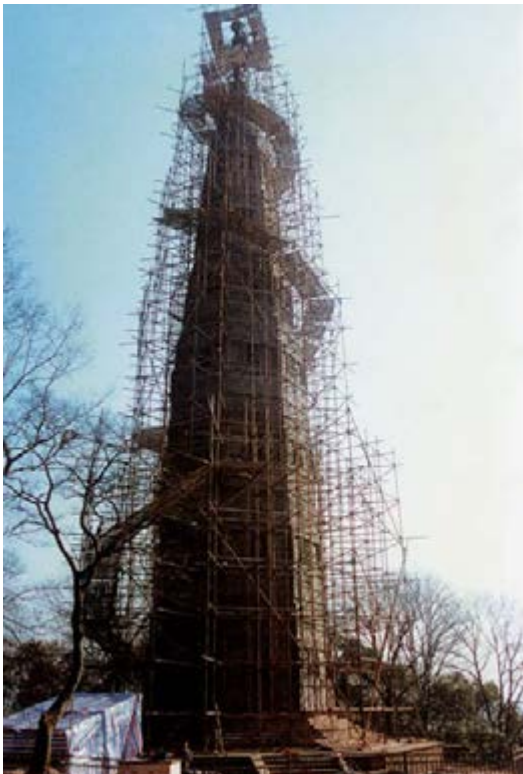
Fig. 4a-10 Reinforcement and maintenance of Baochu Pagoda, photographed in 1997
