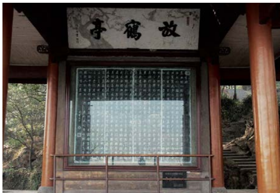
Fig. 4a-17 Protective shelter and railing of Stele of Wu-he-fu, 1986
