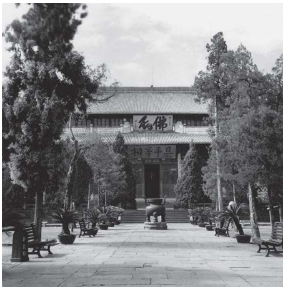
Fig. 2a-119 Historical photograph of the Main Hall of Jingci Temple, photographed during the Republic of China (1912 -1949)
