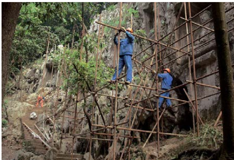
Fig. 4a-14 The 1st-phase protection project of Feilailfeng Peak, photographed in 2005
