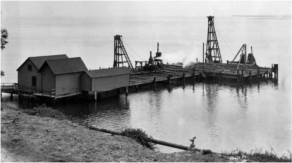
Fort Rosecrans Wharf under construction - c. 1918 ©SDHC 6428.
