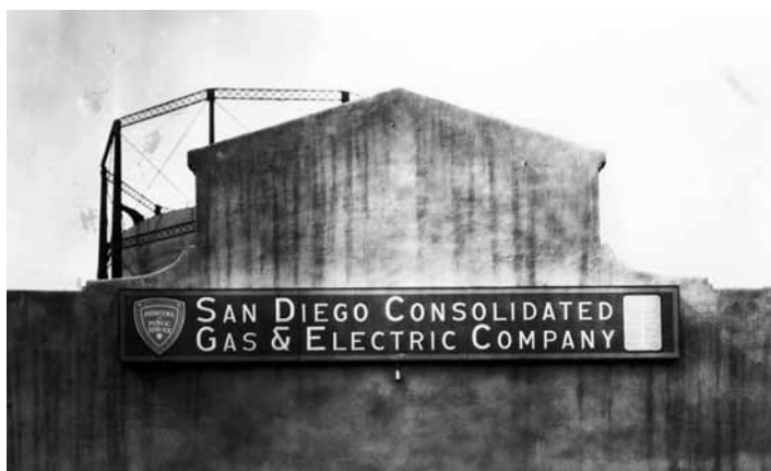
San Diego Consolidated Gas & Electric Company Station ca. 1908. Photo courtesy USD History Archives.
