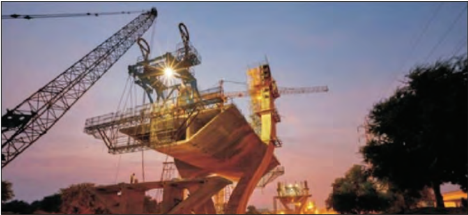
Figure 6.34: Bridge Builder arrangement on pylon-span
