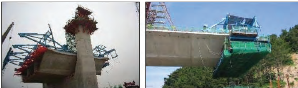
Figure 6.30: Form traveller erection arrangement
