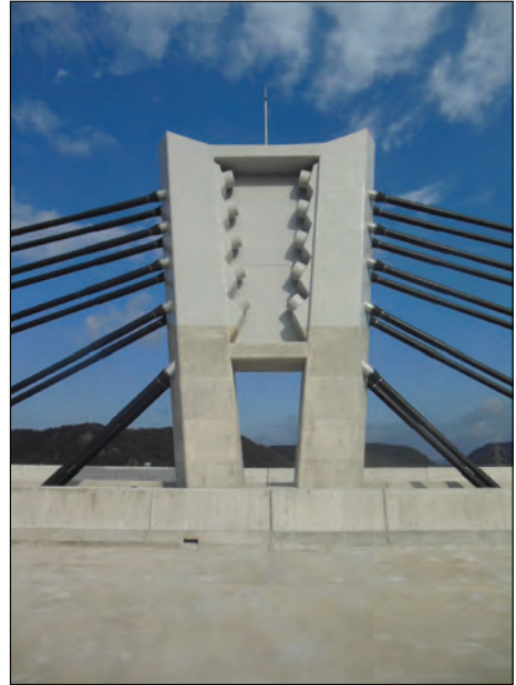
Figure 4.3: Special pylon solution
