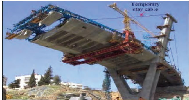
Figure 6.29: Use of temporary stay cables for the construction of Wadi Abdoun Bridge in Jordan
