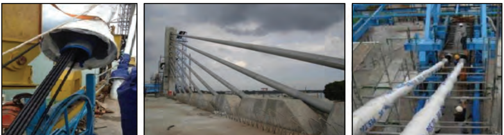
Figure 6.24: stay cable system
