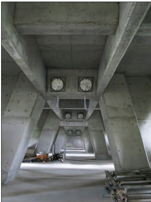
Figure 4.10: Diaphragm of stay cable anchorage in butterfly web
