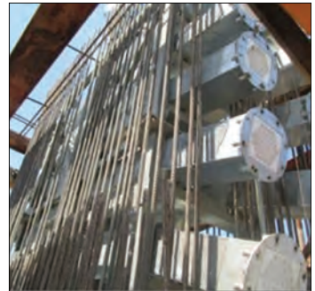
Figure 5.10: View of multitube saddles (copyrights: Freyssinet)
