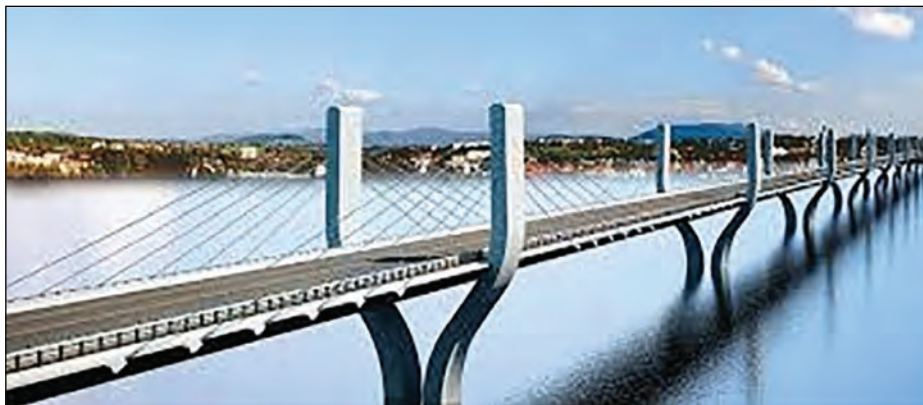
Figure 6.32: Narmada Bridge, Bharauch
