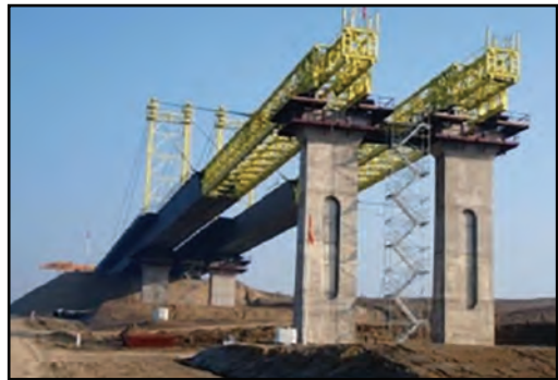
Figure 6.23: Pecs bridges the flat valley of the Szebenyi-river. The straight superstructures were erected by the incremental launching method. The launching nose was supported by stay cables from a temporary tower, located on the deck.
