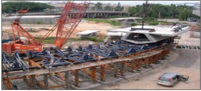
Figure 6.4: Erection of prefabricated segments on scaffolding
