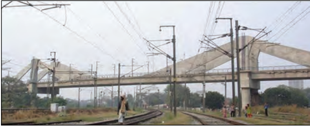
Figure 2.27: Pragati Maidan bridge 46
