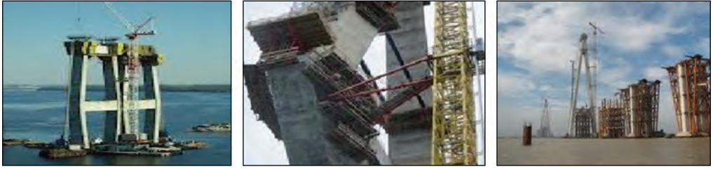
Figure 6.2: Tower crane for pylon construction
