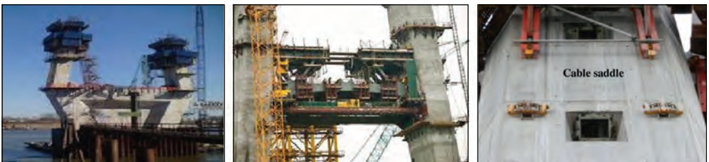
Figure 6.3: Upper pylon construction
