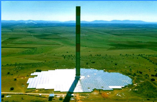
Manzanares 200 m high, 10 m diameter Collector 0.04 sq. km 50 kw, 130 J/kg, 1 Mg/s Spain 1982 to 1989
