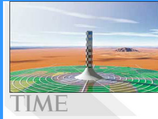
Enviromission 1000 m high, 100 m diameter. Collector 40 sq km 200 MW, 300 tonne/sec Australia / US
