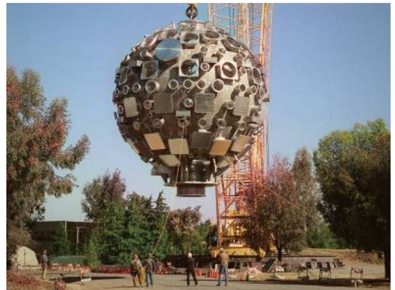
Installation of the target chamber
